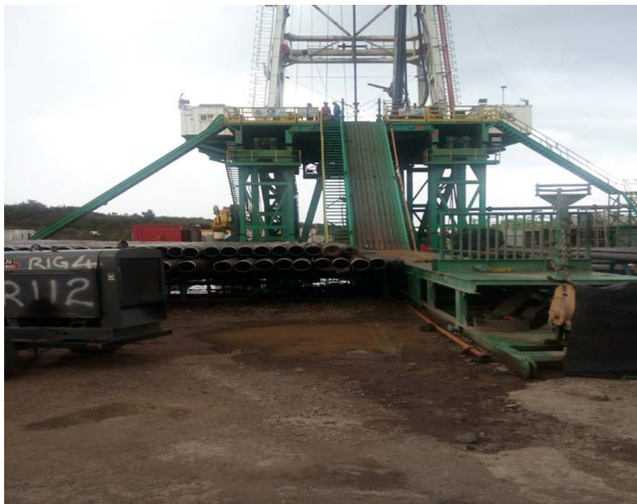
FIGURE 5: Drilling rig with casing joints on the rack
