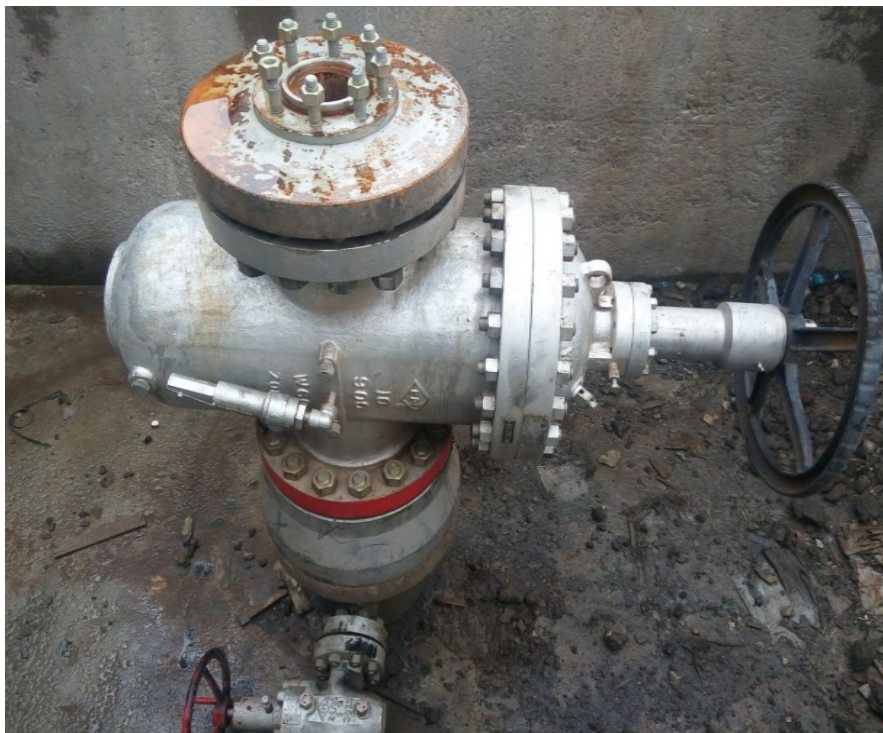
FIGURE 6: Well head assembly
