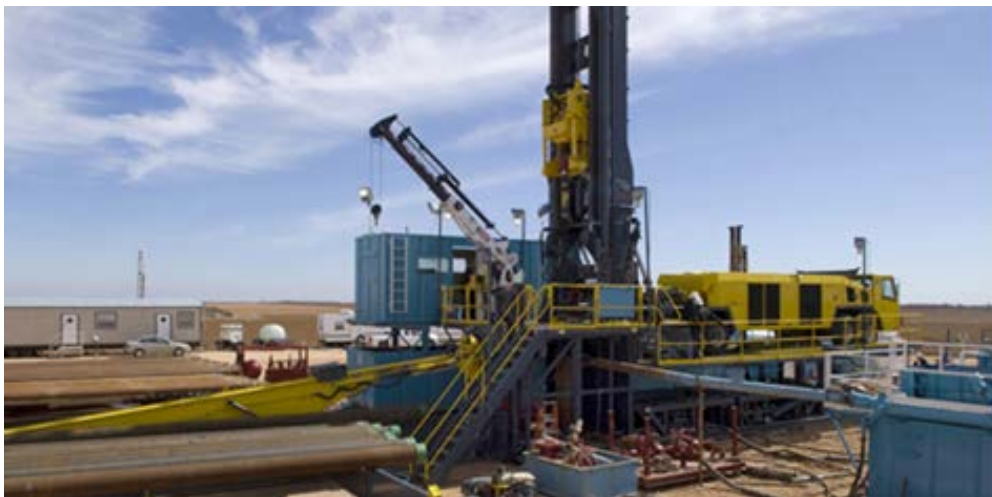
FIGURE 3: Atlas Copco predator rig
