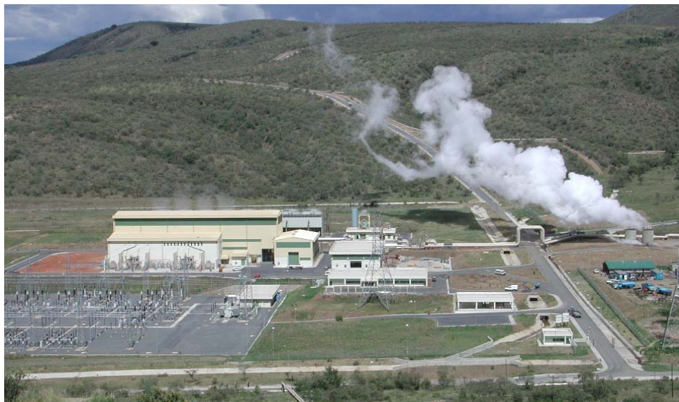
FIGURE 3: Olkaria II Power Station (105 MW)
