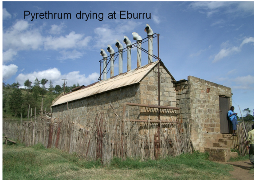
FIGURE 5: Geothermal energy being used by the local community at Eburru for pyrethrum drying Water harvesting
