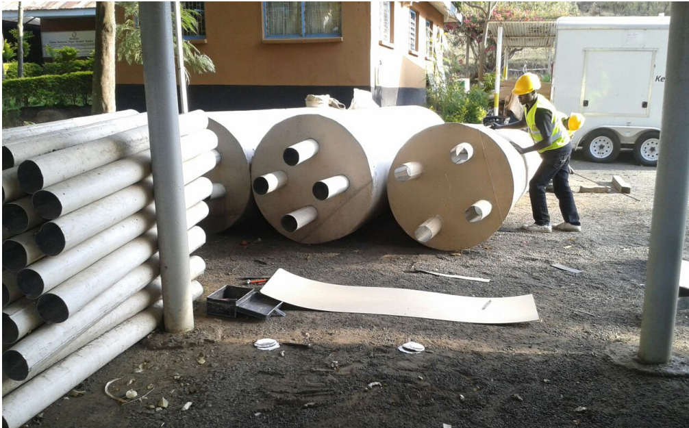
FIGURE 11: Fabrication of steam condensing unit for installation at Eburru
