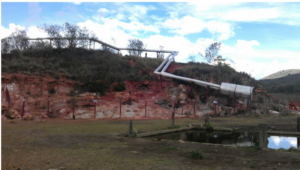
FIGURE 10: Steam condensing unit at the Olkaria Hell's Gate
