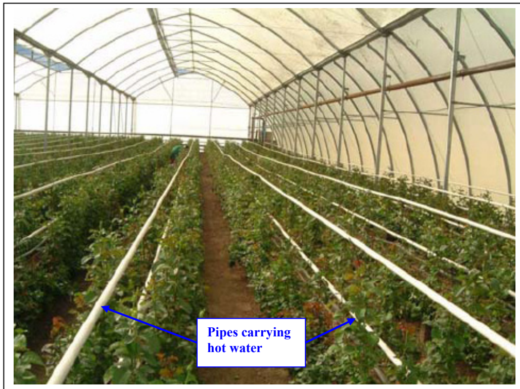
FIGURE 6: Geothermal greenhouse heating at Oserian Company, Kenya.
