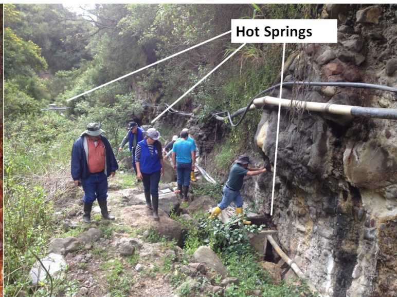
FIGURE 24: Hot Springs entrapped in cement box at Chachimbiro area
