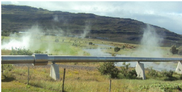
FIGURE 4: Pipeline on the surface (modified from Onyango, 2012)
