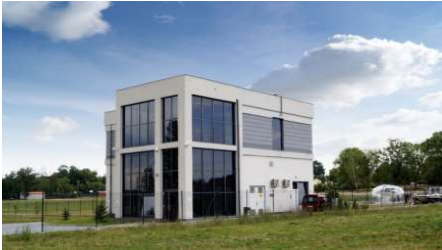
Fig. 2.15. Poddębice geothermal district heating plant – general view
