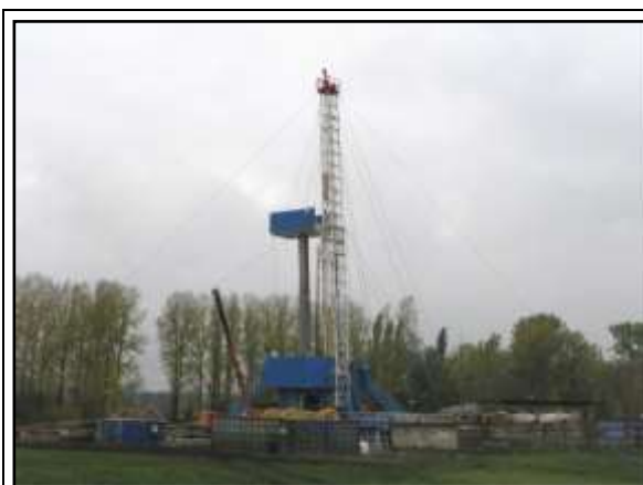
Fig. 2.2. Poddębice GT-2 well drill rig in 2009 (arch. Geotermia Poddębice Ltd.)
