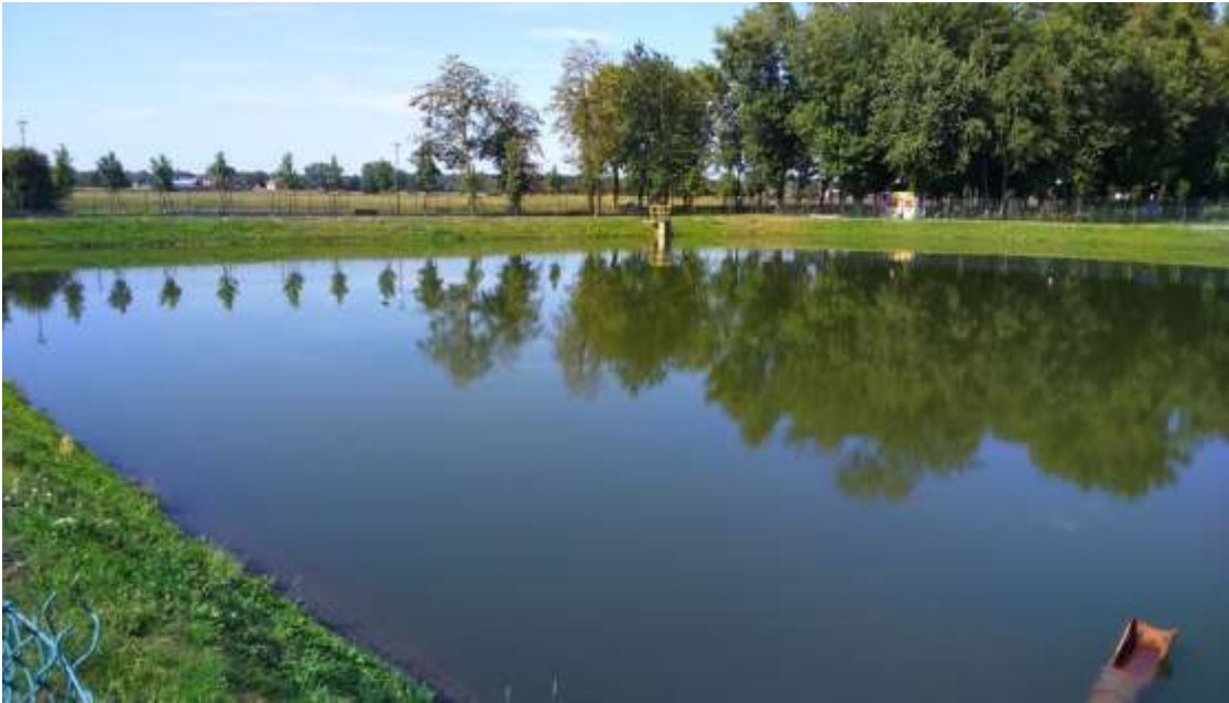
Fig. 2.35. Discharge pond for cooling of return geothermal fluid
