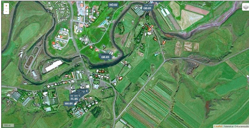
Figure 48. Overview of the wells at Hellisholt and Grafarbakki in the Flúðir System. (NEA's well registry.)
