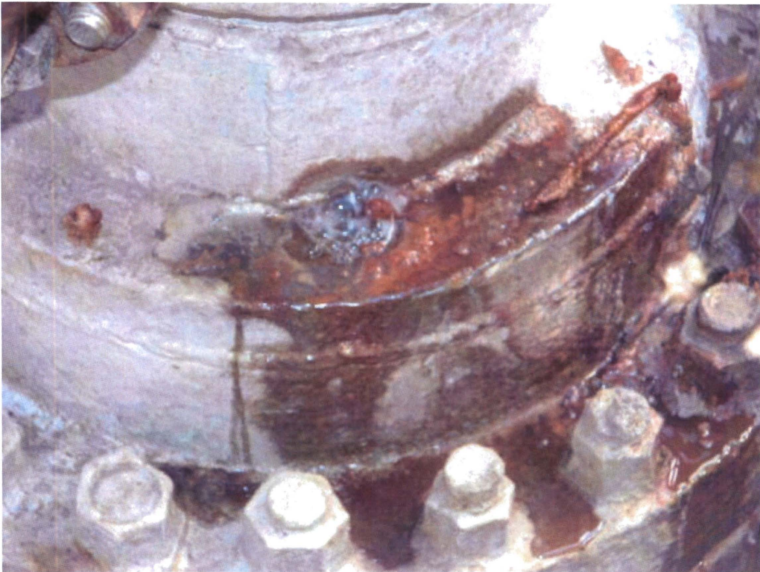
Figure 1. Photograph of the leak on BO-2 wellhead sent to me May 1 (photo H. Correia)
