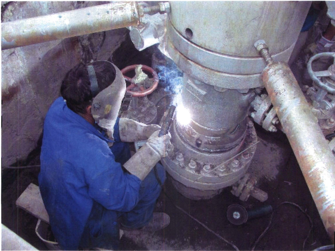
Figure 8. Patch welded in place by a COTUMER welder.
