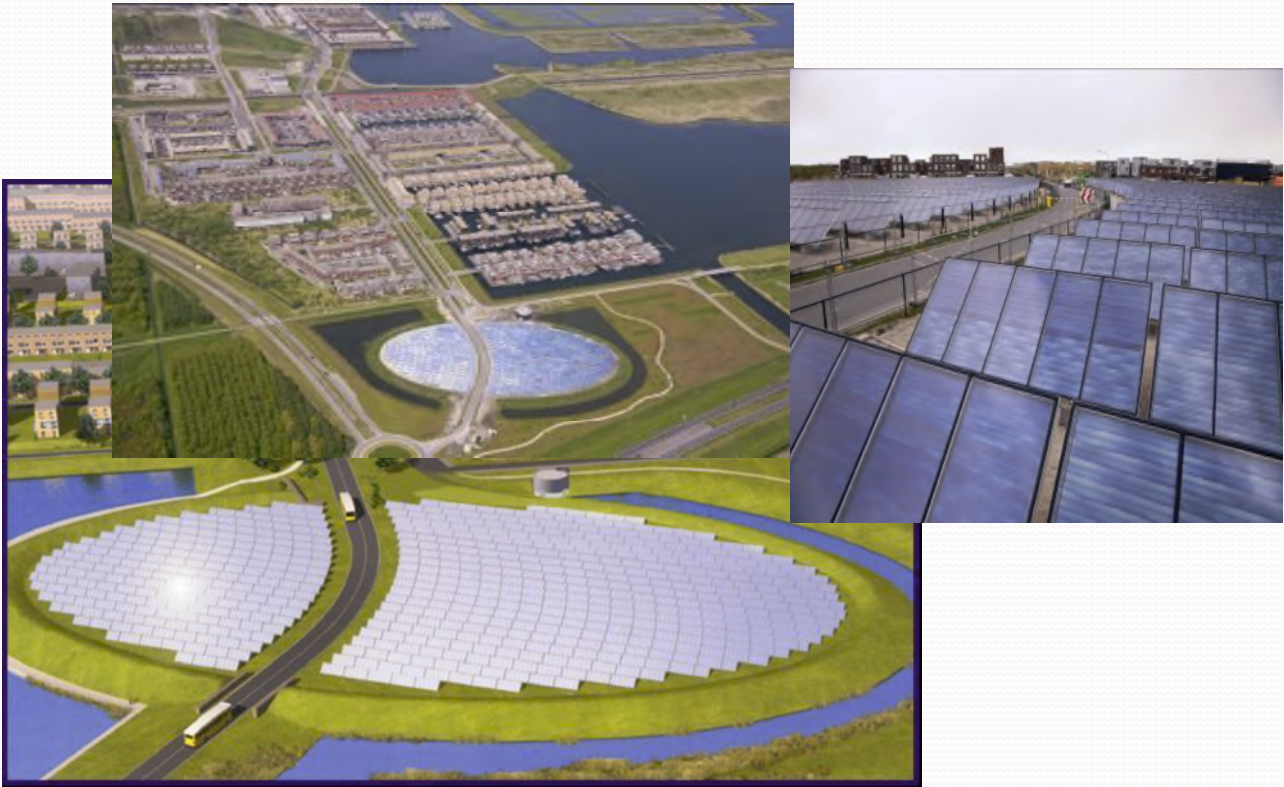
Flat Plate Collectors 7000 m 2 Production 10,000 GJ/y at 75 C
